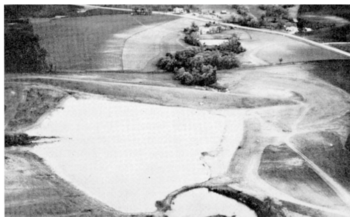
Figure 21.—Aerial view of a floodwater-retarding structure in an area of Stephen-Eddy complex, 3 to 5 percent slopes, eroded.
