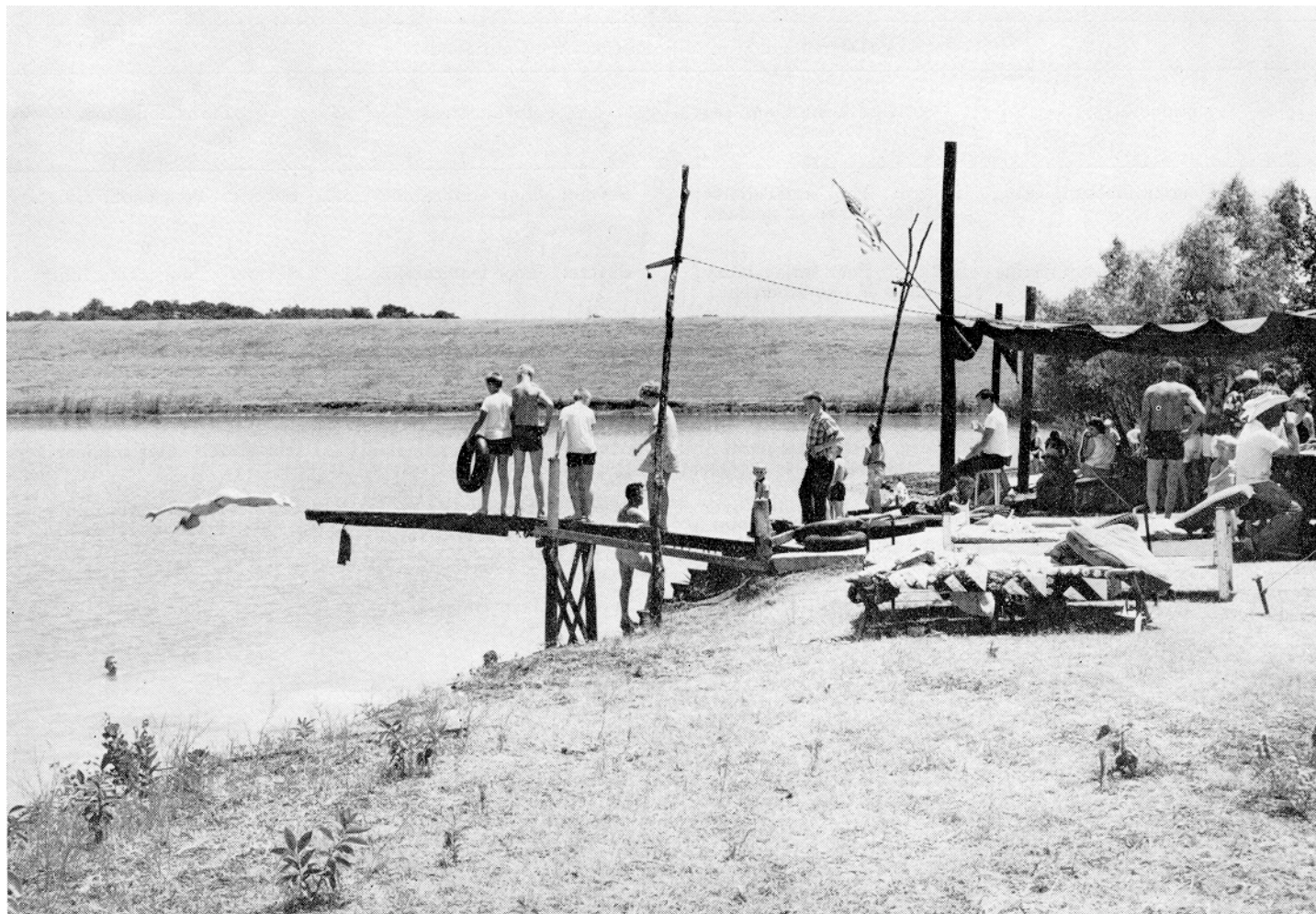
Figure 20. —Part of a floodwater-retarding structure used for recreational purposes. This structure was built in an area of Altoga silty clay, 5 to 8 percent slopes, eroded.
